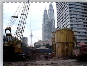
30MN Statnamic Load Test at Kuala Lumpur, Malaysia
